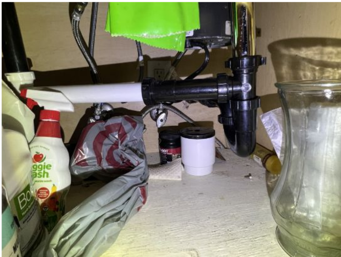
Under Kitchen sink
